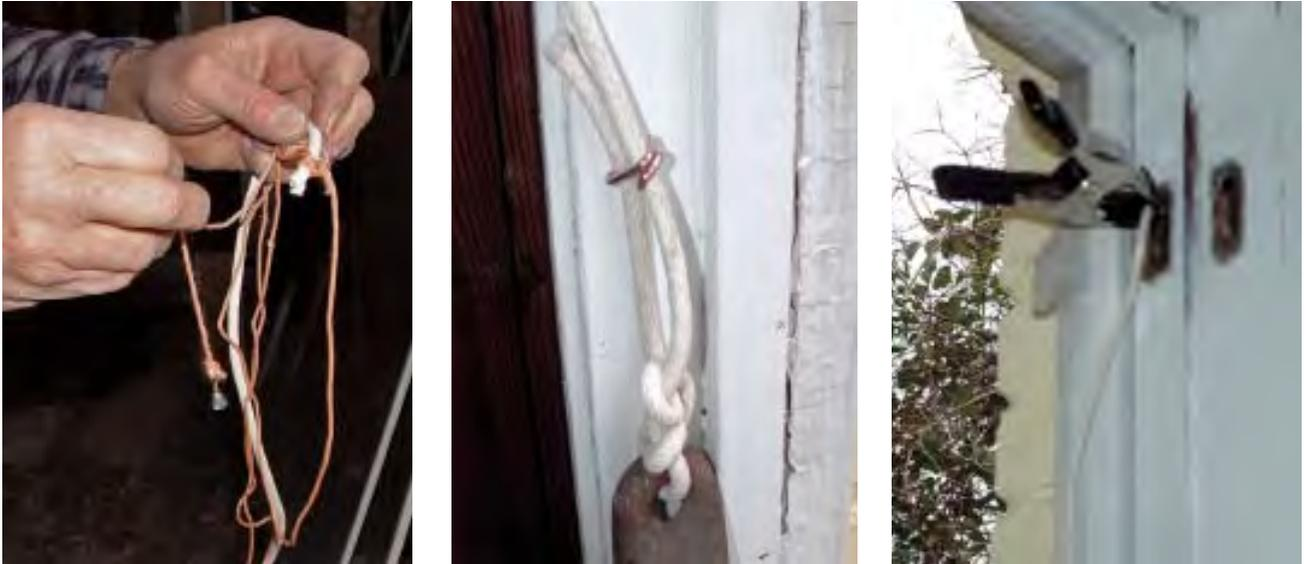
**Figure 5.** A weighted string helps the author fish new sash cord over the pulley and down to the bottom of the weight box (left). He secures the cord to the sash weight with two half-hitches, then captures the excess cord with a hog ring to prevent it from ever getting snagged in the cavity (center). To allow plenty of slack for attaching cord to sash, he pulls the weight to the top of the cavity and clamps the cord (right).
