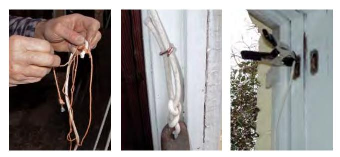
Figure 5. A weighted string helps the author fish new sash cord over the pulley and down to the bottom of the weight box (left). He secures the cord to the sash weight with two half-hitches, then captures the excess cord with a hog ring to prevent it from ever getting snagged in the cavity (center). To allow plenty of slack for attaching cord to sash, he pulls the weight to the top of the cavity and clamps the cord (right).
