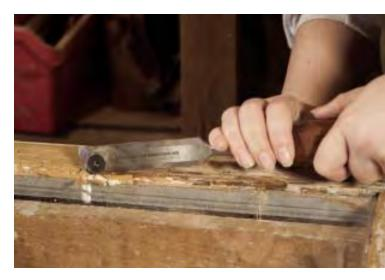
sand all surfaces with 100-grit sandpaper. Then I apply a generous coating of Benjamin Moore's Fresh Start — an alkyd primer suitable for both interior and exterior uses — to all surfaces except the vertical edges. I'm especially careful to fully coat the rebate (the part that holds the glass) because the glazing compound will not bond to bare wood.
