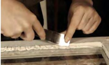
that can be installed from the inside or the outside. I've also had good luck retrofitting sash with weather stripping. Instead of the spring bronze systems that are a nightmare to install, I use an assortment of silicone beads and nylon pyle (brush-type) weather seals; they snap into narrow grooves that I rout into the surfaces of the sash with a specially designed slot-cutting bit (**Figure 4**).
