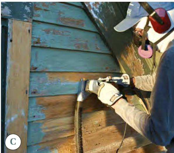
The Paint Shaver's triangular blades (A) can remove unwanted paint from the faces and butts of clapboards at the same time. But in the hands of an inexperienced operator, this powerful tool can easily damage the substrate (B), so it's a good idea to practice on an inconspicuous area. Also, even though the Paint Shaver excels at stripping wide, flat surfaces, it leaves a significant swath of untouched paint in the corners (C) that must be removed by other means.
