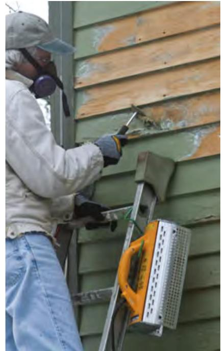
The Speedheater has a multisided profile scraper that allows it to remove paint from moldings (left) as well as flat stock. Unlike high-speed rotary tools that require two hands to operate, it can be used safely on an extension ladder (right).
