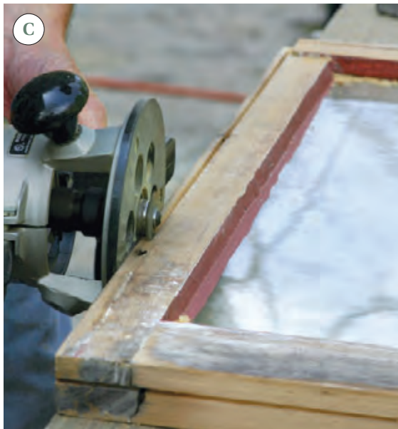
Figure 4. Using a plunge router, the author centers the slot for the bottom tube seal \frac{5}{8} inch from the face of the sash (A); the slot for the meeting-rail seal is centered \frac{3}{8} inch below the top edge (B). The side brush seals are placed as close to the edge as practical — \frac{1}{4} inch (C). Any closer and the thin strip of wood left behind may break off.
