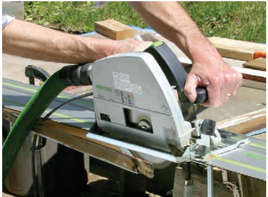
Figure 3. The bottom edge of the sash must be trimmed by about 1/8 inch to account for the thickness of the weather seal (above). After the cut, the end grain gets a treatment of epoxy consolidant to prevent rot infestation (left).
